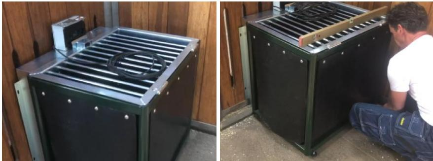
If not, determine which angle is the highest. The other corners can be raised using the adjustable feet. Start with a corner that is next to the highest corner. Place the spirit level between the two corners and turn the adjustable leg clockwise, seen from above, until this side is level.
