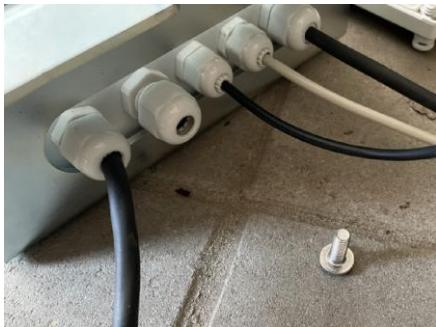
Place the synchronization cable by inserting all four fork cable lugs one after the other through the gland. Both sides of the synchronization cable are equal, so it does not matter which side is used.
