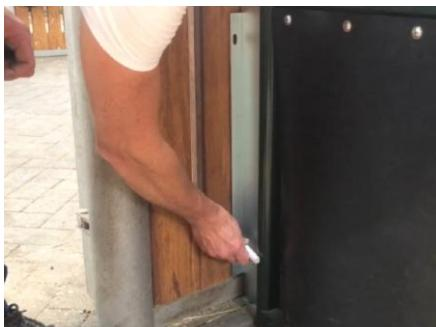
Slide the FeedingMaster away from the wall to drill the holes.
