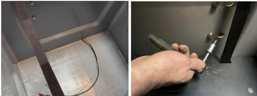
Pull it gently as far as possible while sliding the FeedingMaster toward the wall until the mounting brackets are the against the wall.
