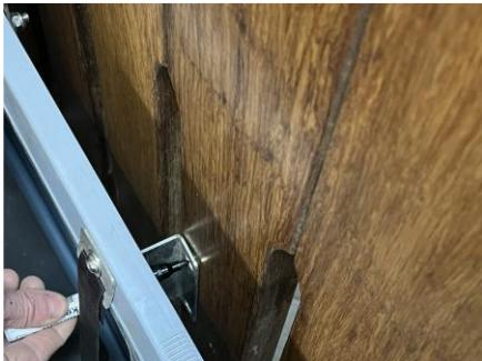
If the hole for the connecting cables is not drilled yet through the wall it can be marked now. Flip the feeding base toward you so that this hole in the lower right rear of the FeedingMaster becomes visible. Insert a felt-tip pen or pencil through the hole and mark the hole on the wall. Gently lower the bottom again.
